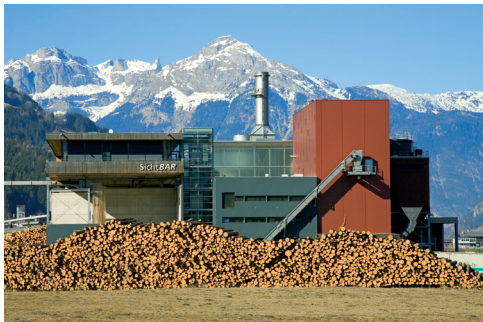
Biomass powerplant "Feuerwerk Binder", Zillertal, Tyrol Architecture: H. Reitter © Günther Richard Wett
